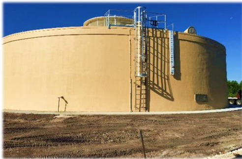
New water tank holds 800,000 gallons
