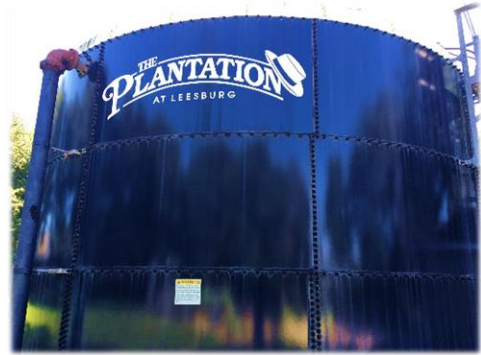
Old tank held 54,000 gallons
